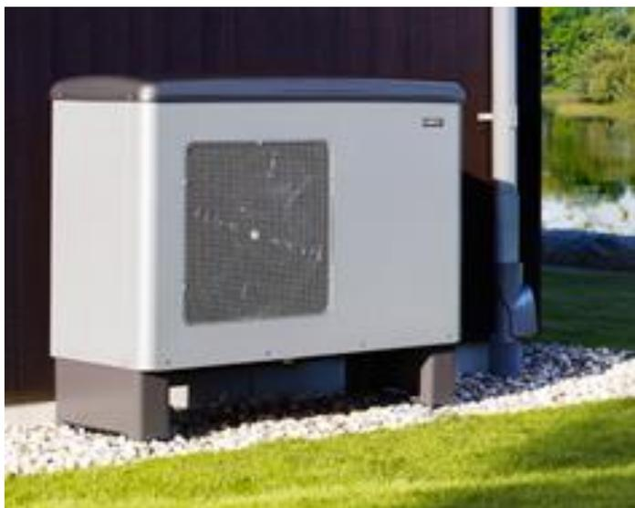
*Air-source heat pump for space heating*
